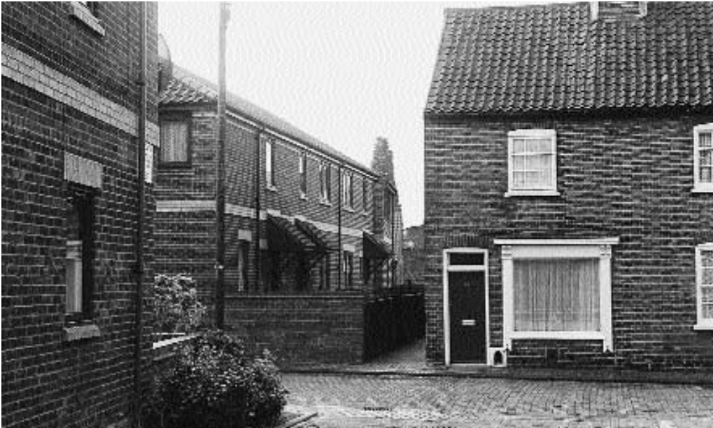
Figure 5.47 Millgate. Completed project.
