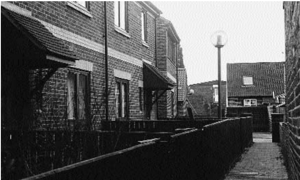
Figure 5.48 Millgate. Completed project.
